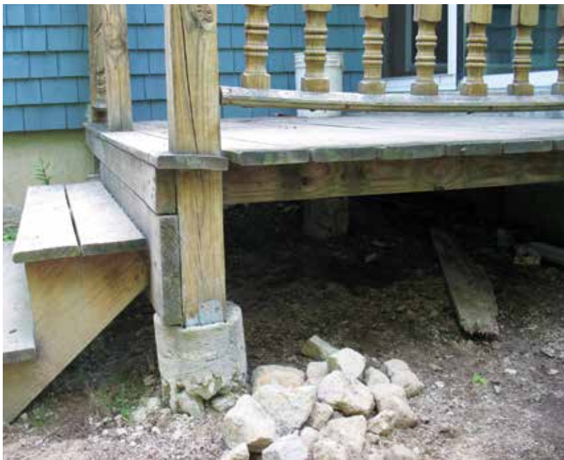
Figure 1. When a pier is angled, deck loads are transferred to the pier's side rather than its bottom, which can cause it to sink. Also note the voids—a result of too many large rocks in the concrete mix—that have weakened this pier.
