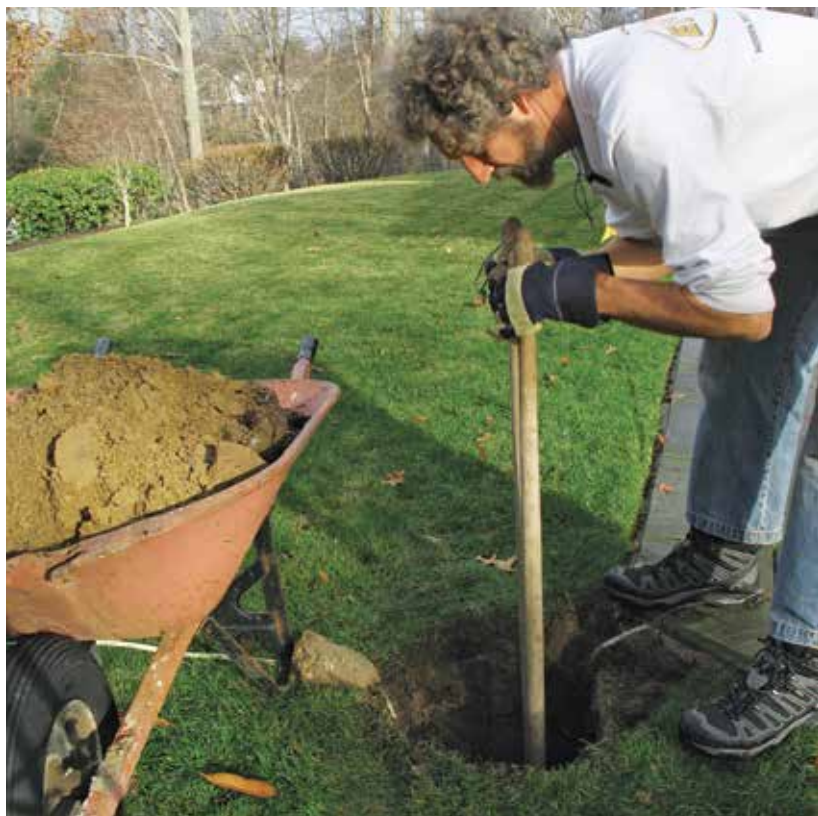
Figure 6. Footings that are sized based on actual deck loads and soil conditions are usually smaller in diameter than when they're sized using prescriptive methods. This makes digging holes for them much easier, especially when frost depths are more than 3 feet below grade.
