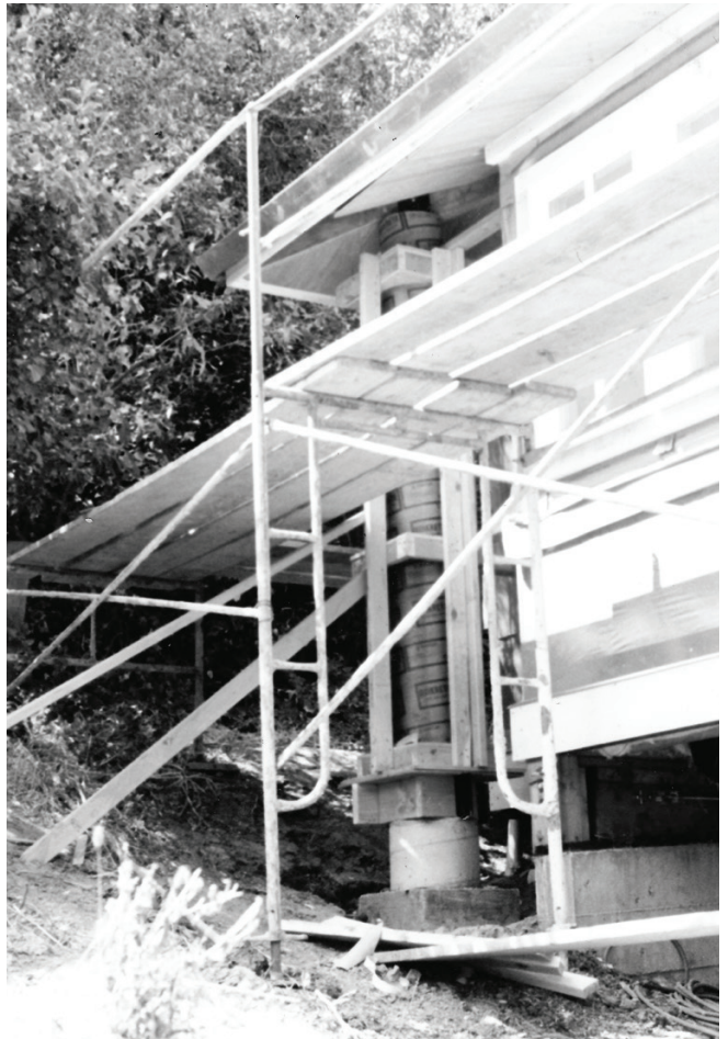
The stepped concrete column (whose formwork is visible behind the scaffolding) was costly to construct for several reasons, including complexity and difficult access. Most impactful, the column was to serve as a prominent finish item, so all forming and concrete installation had to be meticulously controlled.
