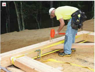
Unity Homes often have a timber-frame component, and this house was no exception. After setting the floor deck panels, the crew assembles a timber-frame bent made from glulam lumber that was cut in the factory (13). Besides adding a distinctive decorative note to the home's interior, the bent supports the main roof. Although cut on CNC machines, all the joints are pegged together in the traditional manner of a timber frame (14).
