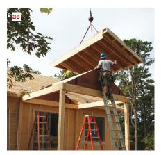
Even the porches are on this house are prefabricated in the factory. Supports for the inner porch walls are part of the foundation pour to avoid the need for a ledger (24). The main porch uses a timber frame to support the roof, but prebuilt gable panels sit on the frame (25). After installing the porch ridge beam, the crew installs the porch roof panels (26).
