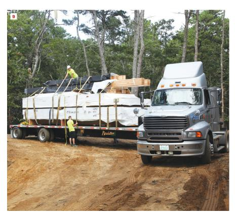
The parts for the house come on big flatbed trailers, shrink-wrapped, labeled, and numbered for assembly (9) After glulam carrying beams supported by posts tenoned into them are dropped into place (10), the crane sets the first-floor deck panels (11). As each floor panel is set in place, the crew draws the panels together with specialized ratchets (12). The panels are then fastened to the sills from below.
