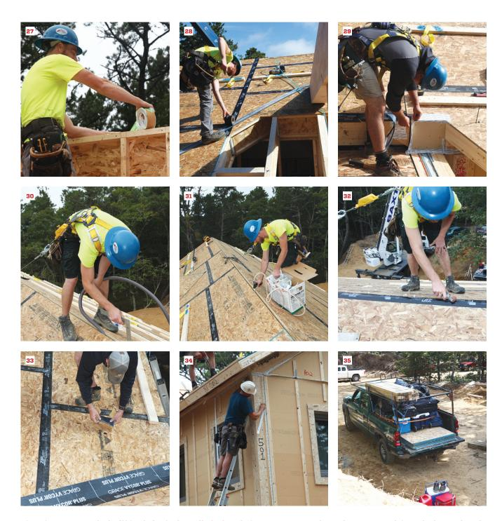
Siga Rissan tape seals the lifting holes in the walls (27), and Zip System tape seals the roof-panel seams (28). A crew member layers the various tapes and gaskets for a crucial wall-roof-deck intersection (29). At the peak, backer rod fills the gap between panels (30), followed by expanding foam (31) and Zip tape (32), which also seals roof-panel holes (33). Siga Wigluv tape air-seals the wall-panel intersections (34).
