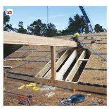
After attaching gasket material to the top plates of the walls, the crew sets the gables (19). Roof panels have an integral lip that fits into a groove on the top of the bent beam (20). Chainfalls on the lifting straps hold the panels at the proper angle (21). After installing the intersecting roof beam (22), the crew staples gasketing to the roof in preparation for the next roof panels (23).
