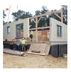
Specialized gaskets are attached to the floor panels (15) before the wall panels are dropped into place (16) to air-seal this critical joint. Note that each panel is fully insulated and comes with an interior 2x3 wall for running utilities. As each panel is set and braced, the crew attaches the gasket material to the corner of the panel where it meets the adjoining wall panel (17). After raising the timber-frame bent, the crew continues to stand the walls around the house (18).
