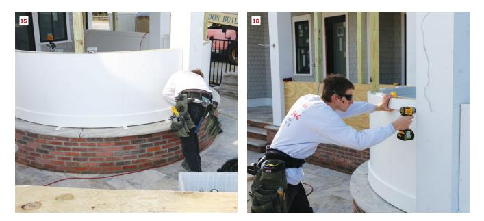
For the rails on the outside curve of the knee wall, the crew installs the same dimension top and bottom rails as on the inside. After cutting the bottom rail to length, a crew member screws it through the flat panel and into the knee-wall framing, working from one side to the other **(15)**. As with the sheet stock, one end of the 1x4 top rail can be clamped in place while a crew member secures the rail in place with stainless steel screws **(16)**.
