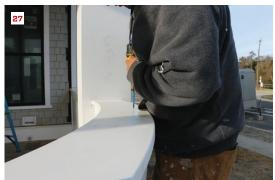
To lay out the location of the intermediate post, the crew snaps a line from the pivot point through the centerline of the arc (24) and marks the post location (25). After dividing the top cap into two pieces by cutting along the centerline, a worker uses a jigsaw to cut out the post **(26)**, then screws the cap to the knee wall (27).
