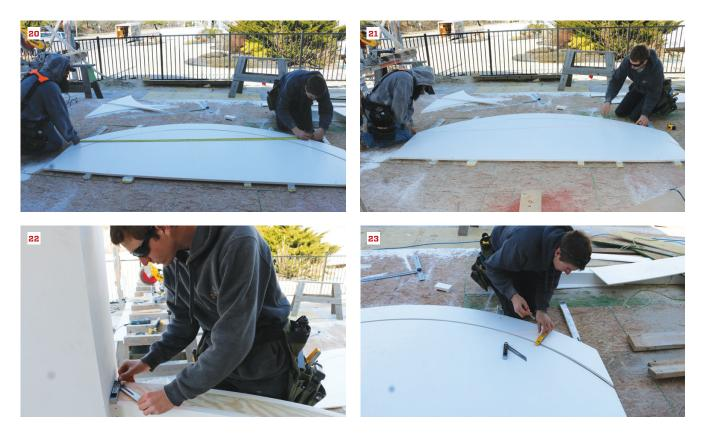
After measuring a straight line between the posts for each arc, the crew transfers the measurement to the radiused cap (20) and snaps a chalk line between the end points (21). Having snapped the same line on top of the knee wall, a crew member measures the angle between the snapped line and the post (22). He then transfers the angle to the radiused stock and draws straight lines for the end cuts of the cap (23).
