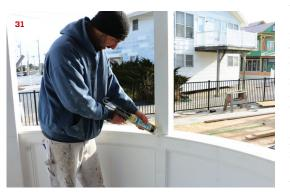
PVC panel molding completes the paneling outside (28) and in (29). The crew wraps the intermediate posts in PVC using the same method described in "PVC Miter-Fold Post Wraps" (Jul/16). The PVC wraps nail directly to the 4x4 posts **(30)**. The final step is caulking all the joints, filling the fastener holes, and prepping for the painter **(31)**.
