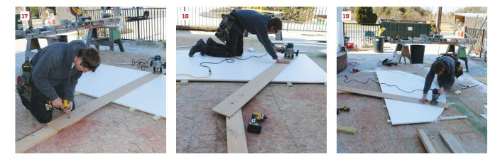
The cap for the curved panel walls is cut from <sup>3</sup>/4-inch-thick PVC sheet stock. With the router mounted on the same trammel arm that he used before, a crew member first sets the radius for the outside of the curved cap rail and drives a screw to secure the pivot point (17). Making multiple progressively deeper passes, he cuts the outside radius for the cap rail (18). After resetting the pivot point, he makes the cut for the inside radius of the cap rail (19).
