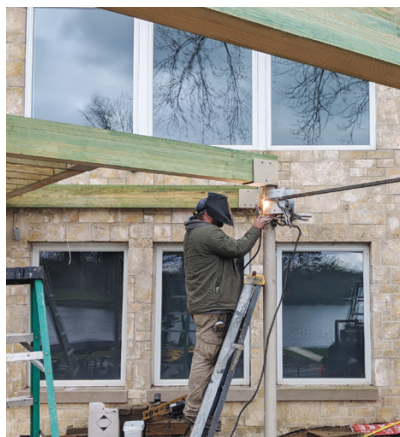
Custom-fabricated brackets were welded to the steel columns to support dropped beams (above left). Cantilevered joists were then installed to create the shape of the guitar body (above center). Extensive blocking was also needed to execute the elaborate inlay required to create the guitar design (above right).
