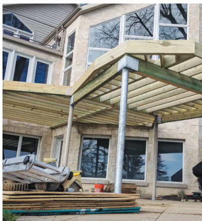
Custom-fabricated brackets were welded to the steel columns to support dropped beams (above left). Cantilevered joists were then installed to create the shape of the guitar body (above center). Extensive blocking was also needed to execute the elaborate inlay required to create the guitar design (above right).
