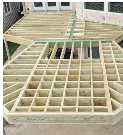
Custom-fabricated brackets were welded to the steel columns to support dropped beams (above left). Cantilevered joists were then installed to create the shape of the guitar body (above center). Extensive blocking was also needed to execute the elaborate inlay required to create the guitar design (above right).
