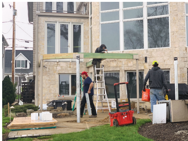
The steel columns, stainless steel spiral staircase, and custom-fabricated handrails from the original deck (above left) were repurposed on the new deck, which needed additional steel columns and PT glulam beams (above right).
