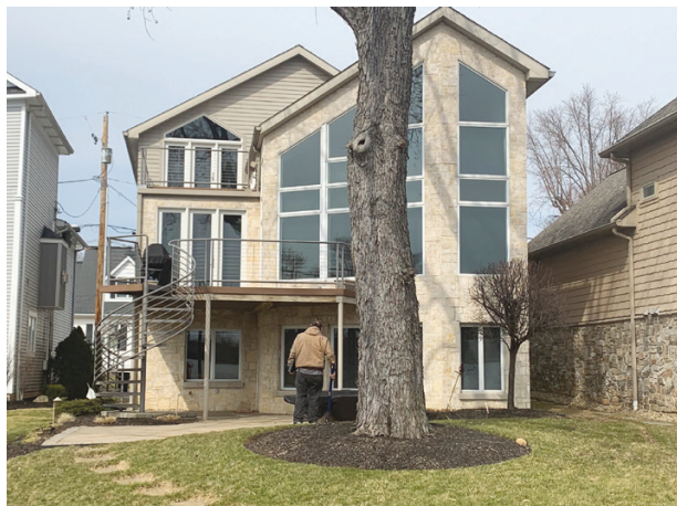
The steel columns, stainless steel spiral staircase, and custom-fabricated handrails from the original deck (above left) were repurposed on the new deck, which needed additional steel columns and PT glulam beams (above right).
