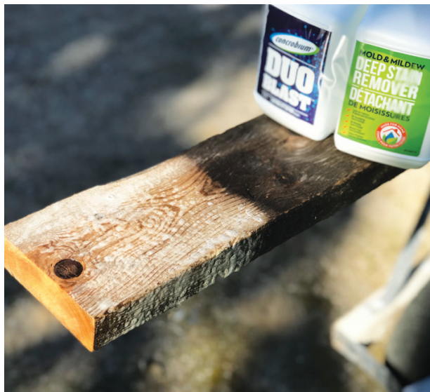
Figure 3. After removing the old finish, you may need to use a deck brightener to return color to weathered, gray decking. Some brighteners contain oxalic acid and need to be neutralized afterward, but the author recommends Duo Blast, which isn't harmful to plants and requires only a water rinse.
