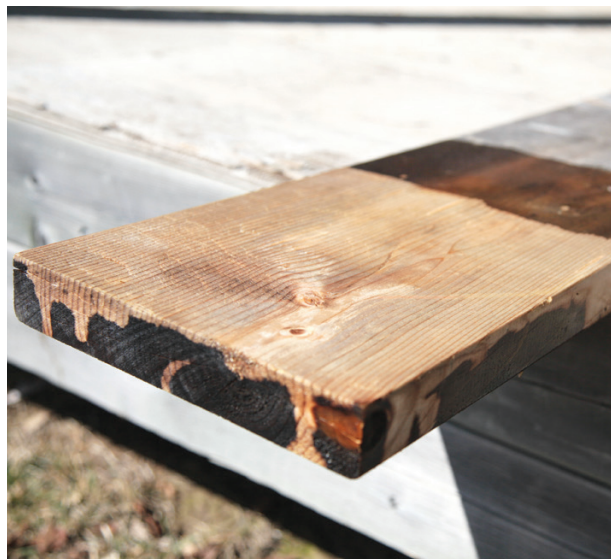
Figure 3. After removing the old finish, you may need to use a deck brightener to return color to weathered, gray decking. Some brighteners contain oxalic acid and need to be neutralized afterward, but the author recommends Duo Blast, which isn't harmful to plants and requires only a water rinse.
