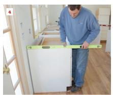
Common scribes are fitting baseboard to a floor (1), scribing a cabinet to a wall (2), and scribing to an irregular surface (3). Shim cabinets level before scribing (4).
