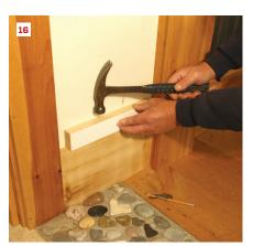
The photos above illustrate the process of scribing a baseboard section to the irregular surface of randomly shaped pebbles (see photo 3 on page 7 for the finished scribe). The steps are described starting on page 8.
