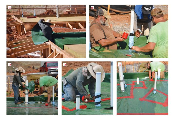
The crew placed a 15-mil polyolefin vapor barrier (Perminator from WR Meadows) across the slab and down into and up out of the footing trench (11). They wrapped the conduit and pipe that penetrated the poly with more poly, tape, and sill sealer (12-15). Later, they would remove the sill sealer and seal the gap using liquid-applied flashing.
