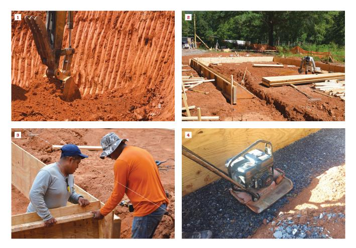
The author had to borrow red clay from off site (1) to create a strong sub-base for the slab. Trenches for the turndown portion of the slab were dug around the perimeter, then the foundation crew started by running 2-foot-high exterior forms around the perimeter (2, 3). Gravel was placed in the bottom of the trench and leveled (4).
