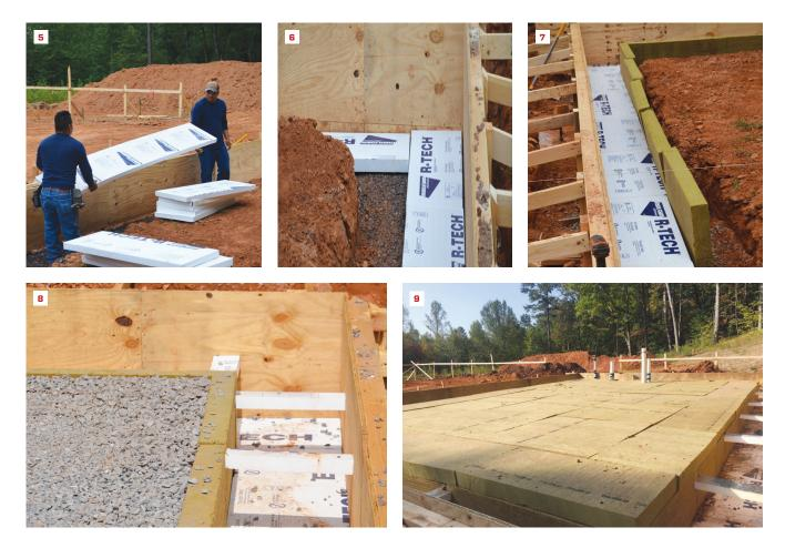
The crew set R-Tech Type IV polystyrene insulation in the bottom of the footing trenches on top of the gravel (5, 6). They placed Rockwool Toprock DD insulation on the inside face of the trench (7), placed gravel in the sub-slab area, and braced the Toprock DD back using small pieces of polystyrene (8). Finally, they filled in the interior of the slab with Toprock DD (9).
