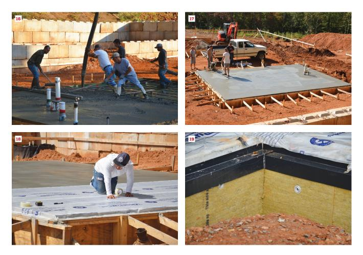
The author specified a 3,000-psi mix placed at a slump of 4 to 5 inches **(16)**. Bleed water had to evaporate completely before the slab could be power-troweled **(17)**. After finishing, the crew applied protective plastic over the slab to maintain good curing conditions **(18)**. On a later project, the author specified a termite shield over the mineral-wool insulation **(19)**.
