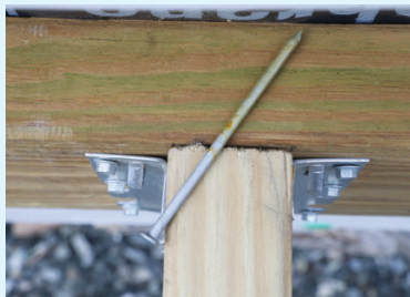
As gap size between the joist and ledger increases, the holding power of diagonal shear nails decreases, reducing the joist hanger's uplift capacity.
