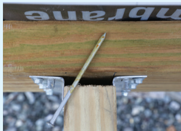
As gap size between the joist and ledger increases, the holding power of diagonal shear nails decreases, reducing the joist hanger's uplift capacity.
