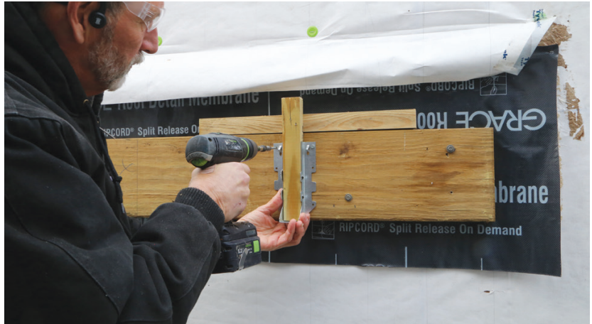
Figure 5. The author prefers to install joist hangers prior to hanging joists, using a site-built T-jig to quickly and accurately place the hangers. When using this method, be sure that the joists are uniformly sized.
