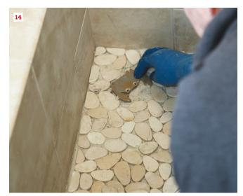
I applied it, there were a few ridges in the surface. So the next day, when the Laticrete was set up but still not fully cured, I used a sharp chisel to cut off the ridges and make a flat surface (10).
