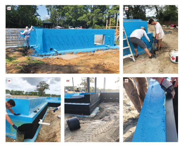
On this project, the CMU walls were sprayed with Poly Wall Home Stretch liquid waterproofing membrane (17), then covered with Arroyo dimple-mat drain board glued to the walls with Quick Grip spray adhesive (18, 19, 20). The tops of the walls are capped with aluminum flashing bedded in sealant (21), while masonry shelves are flashed with Home Stretch detail tape.
