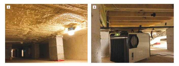
Spraying the underside of this concrete porch floor with foam insulation is a necessary step in turning the crawlspace beneath into conditioned space (1). With a slab over the crawlspace's vapor barrier and with lighting and dehumidification, the space is easier for the homeowner to maintain (2).
