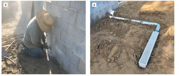
A worker preps the interior of a CMU wall to accept a layer of rigid foam by grinding off mortar drops and other irregularities (3). Installing drains prior to placing the vapor barrier and pouring the slab helps avoid trapping water underneath the house (4).
