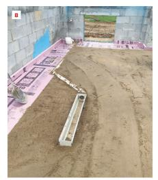
A crew member preps the perimeter of the crawlspace for a continuous 2-foot-wide layer of 2-inch XPS foam (5). Then 6-inch-wide XPS strips are fastened to the walls, with the top edge of the foam aligned with chalk lines marking the top of the slab (6, 7). After the drains and perimeter foam are in place, the sand base is raked smooth in preparation for the vapor barrier underneath the slab (8).
