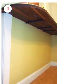
neath. We then routed slots in the bottom (3) and installed the top, using silicone to seal the connection between the wood and steel. A few coated screws driven up through the steel hold it in place (4), where it seems to float above the floor.
