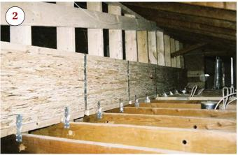
a structural engineer to make sure we were on the right track. Now, as long as we're dealing with the ordinary attic loads found in ranches, we size the engineered beam and metal connectors from the manufacturers' design guides.
