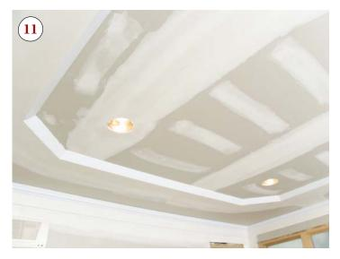
takes texture and paint and gets finished with the ceiling for a seamless appearance. He prices the average soffit at about \$10 per linear foot, based on the room's perimeter dimensions. — *Dave Holbrook*
