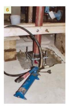
at the top to prevent accidental spills) provided a simple means of monitoring the load transfer. As soon as I felt some slack in the shoring post, I knew the permanent column was preloaded. At that point, all we had left to do was tighten up the bottom nuts under the base plate, place top nuts on the bolts, and release and remove the jack.
