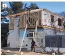
The house before a pop-up addition was built (1). Working outside over existing living space in winter and maintaining 6-foot social distancing, carpenters removed existing roof framing (2), while electrical subs working closer together wore masks rewiring ceiling lights (3). The home was tented off as necessary (4). Demo began on a Monday and the new pop-up addition (5) was shingled by Saturday afternoon. Access to the second-level work area was by ladder only at this stage.
