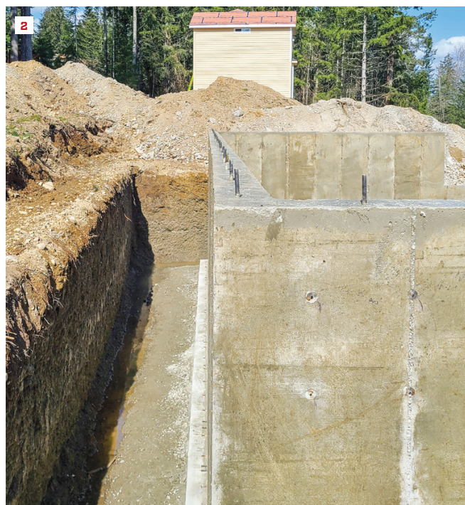
The blue AnchorMate bolt holders (1) simplify the placement of anchor bolts and ensure consistency (2) that in turn simplifies the alignment of the mudsill later.
