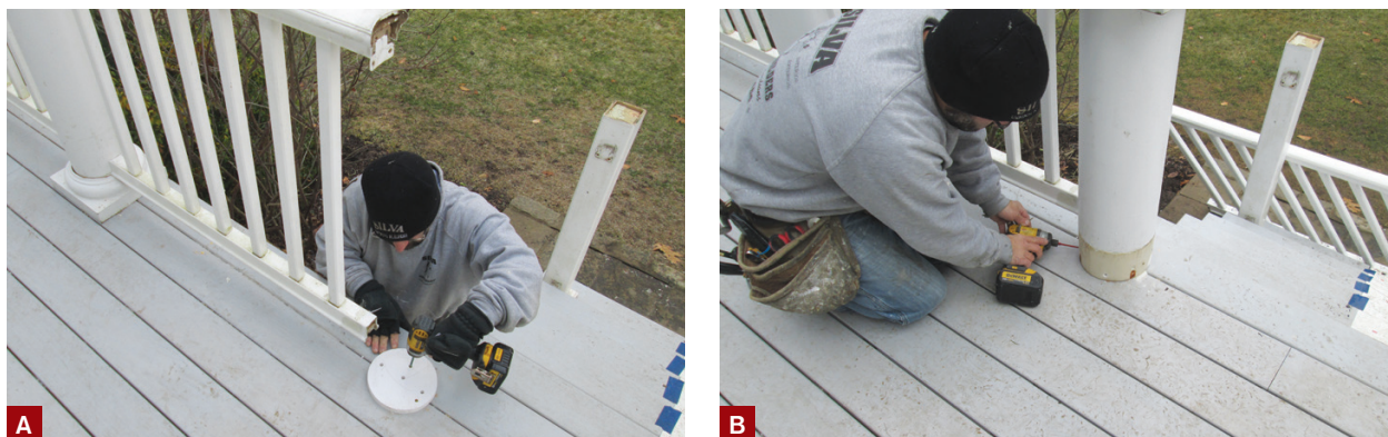
Figure 4. The author cut PVC plugs sized to fit inside the bases of the columns and screwed them to the decking (A). This ensured that the columns would be reinstalled in their original locations (B) and that the railings could be reused.
