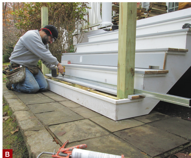
Figure 2. The author reframed the front stairs, cutting new stringers and installing a new dropped header to help support them (A). New 5/4x6 deck boards were face-screwed to the framing after the PVC skirts and risers were installed (B).
