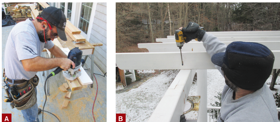
Figure 4. The author cut PVC plugs sized to fit inside the bases of the columns and screwed them to the decking (A). This ensured that the columns would be reinstalled in their original locations (B) and that the railings could be reused.
