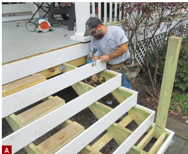
Figure 2. The author reframed the front stairs, cutting new stringers and installing a new dropped header to help support them (A). New 5/4x6 deck boards were face-screwed to the framing after the PVC skirts and risers were installed (B).
