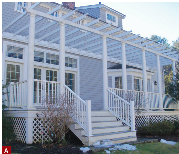
Figure 1. While the original porch framing was sound, the worn and weathered decking needed replacement (A). Part of the repair strategy was to retain the stringers for one set of stairs but pour a new landing pad to support them (B).
