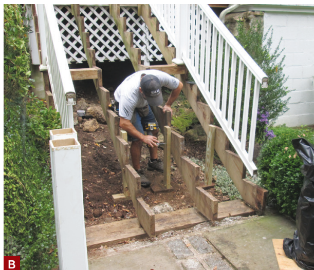
Figure 1. While the original porch framing was sound, the worn and weathered decking needed replacement (A). Part of the repair strategy was to retain the stringers for one set of stairs but pour a new landing pad to support them (B).
