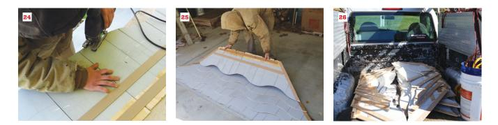
After the strips for four or five courses have been assembled, a worker cuts the waves on each section with a jigsaw (24). Laying the shingle strips out on the shop floor allows them to be checked for mistakes prior to delivery to the jobsite (25). On this job, all the assembled shingle strips that were needed to complete the four gables fit into the back of a pickup truck (26).
