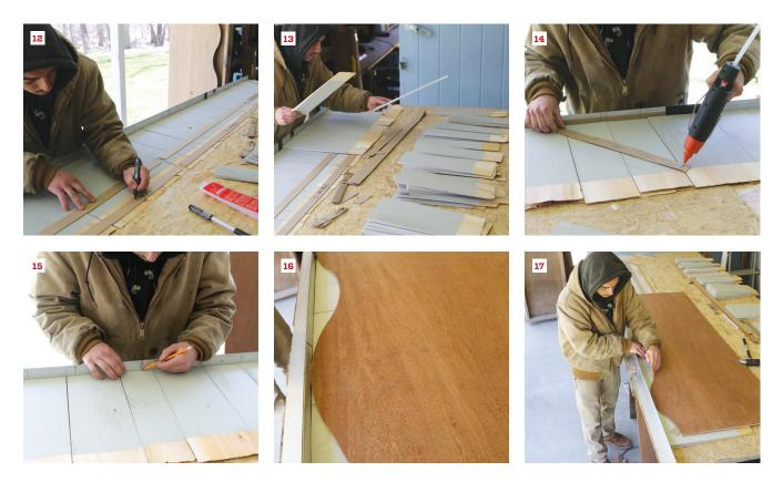
The three collated shingle strips making up the course are labeled with a course number and as a center, left-, or right-hand strip (12). The first wave-course shingles are placed directly over the base course, with the joints offset a minimum 1½ inches (13), and shims are glued on the diagonal to match the rake (14). Working from the centerline marked on the straightedge (15) and the first wave offset line marked on the template (16), a worker draws the pattern on the shingles (17).
