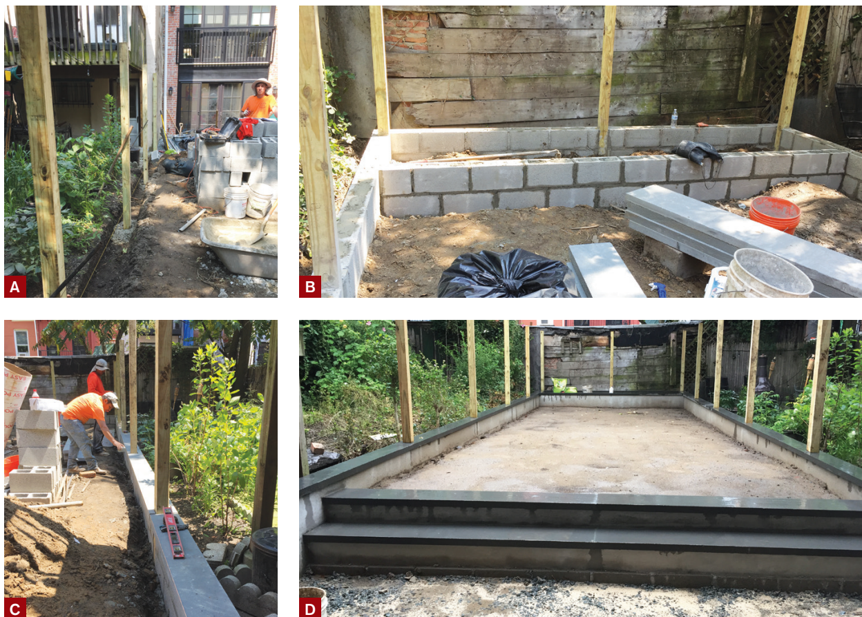
Figure 2. The 4x4 posts for the perimeter fence were set in 3-foot-deep holes that were then filled with concrete (A). Over a compacted gravel base in the bottom of the trench, masons laid up a short CMU wall around the perimeter of the yard, as well as a wall to create a small planting bed at the back of the yard (B). The walls were capped with bluestone (C). Bluestone treads were installed on the steps leading down to the lower level near the house (D).
