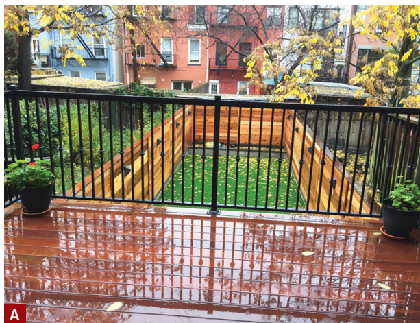
Figure 5. The ipe deck was finished with a custom-fabricated iron railing (A) and looks out over the compact backyard, which serves as a low-maintenance play area for the young family (B). Surrounded by a fence composed of red cedar boards, the backyard is covered with artificial turf instead of grass.
