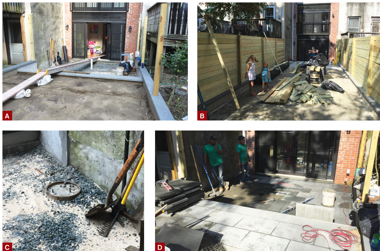
Figure 3. All materials had to be transported by hand from the curb at the front of the house to the backyard through the brownstone townhouse (A). Around the exterior of the perimeter fence, \frac{5}{4} \times 6 pressure-treated decking was installed horizontally up to the maximum 66-inch height of the fence (B). Footings for the deck's two 6x6 support posts were poured (C) prior to the installation of the bluestone paver patio in the lower area (D).
