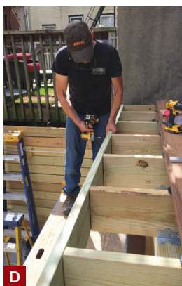
Figure 4. Before the ledger for the new deck could be installed, the opening between the two solid brick walls was padded out with solid 2-by blocking and a PVC shim (A). The ledger was fastened to the framing under the door opening with lag bolts and to the solid masonry wall with epoxied expansion bolts (B). The rest of the rectangular 9-foot-by-12-foot deck was conventionally framed with PT 2x10s (C) cantilevered over a dropped triple 2x10 beam (D).
