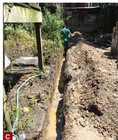
Figure 1. Measuring just 15 feet wide, the overgrown backyard was bordered on two sides by an old cyclone fence (A). After removing it, workers removed the sod and brought in materials to build a short CMU retaining wall around the yard and a perimeter fence (B). With no access for machinery, the trench for the perimeter fence was dug by hand (C).
