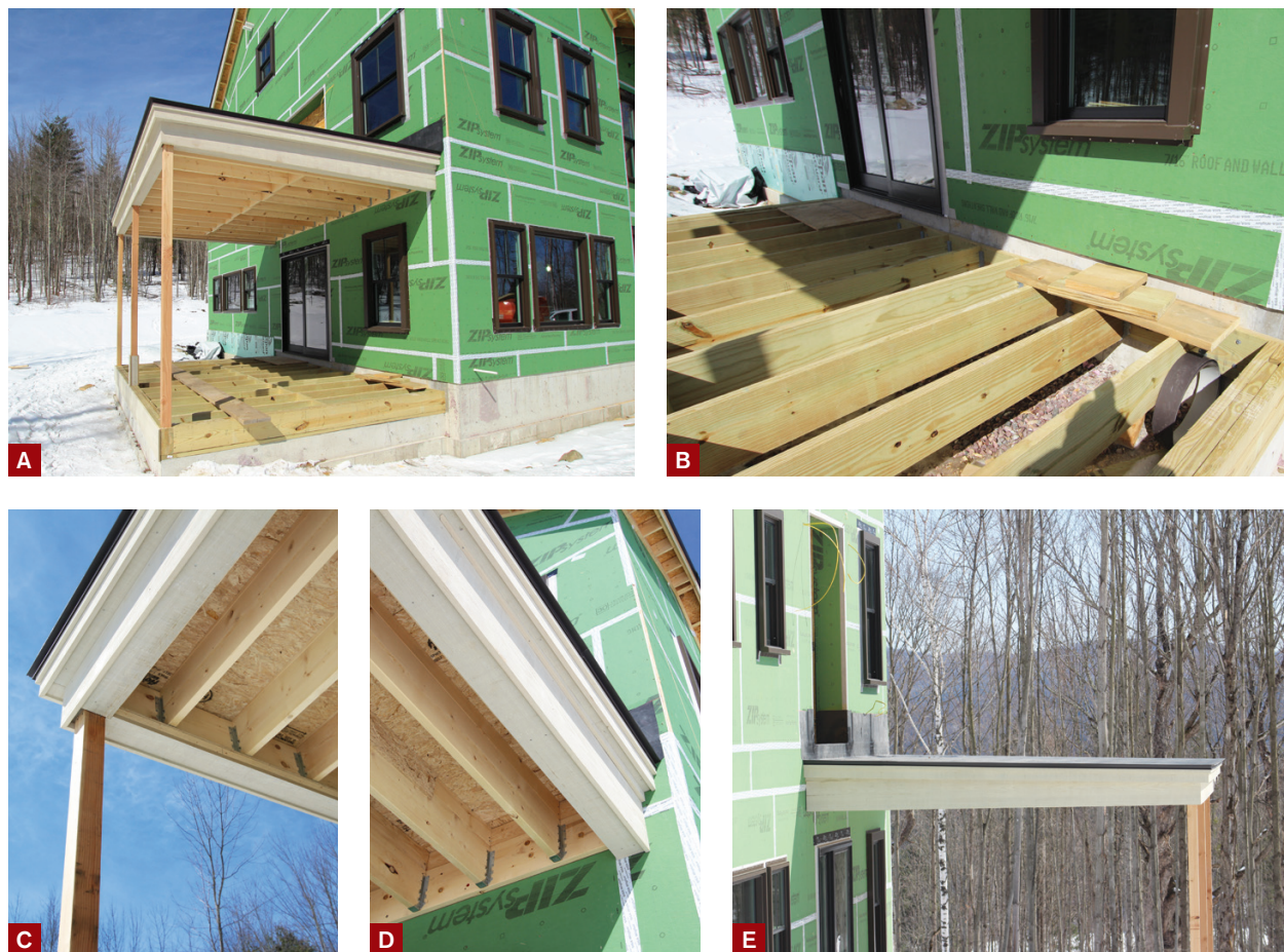
Figure 1. The screened porch was conventionally framed like a deck with pressure-treated lumber but supported by a poured concrete stem-wall foundation rather than posts or piers (A). The deck ledger was bolted to the home's concrete foundation with wedge anchors (B). Tapered rippings added to the ceiling joists (C, D) created the pitched roof deck (E).
