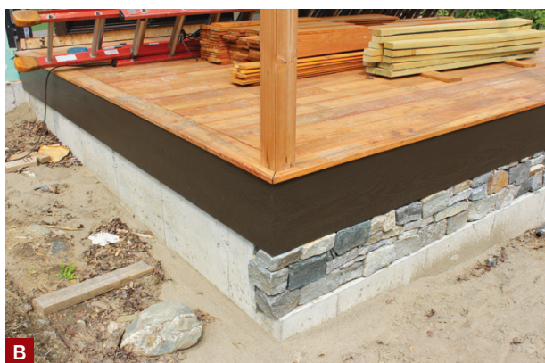
Figure 3. The porch fascia, posts, and eaves were trimmed with Boral TruExterior trim, which is made with fly-ash, a coal combustion by-product, mixed with polymers (A). The porch foundation received a fieldstone veneer finish (B).
