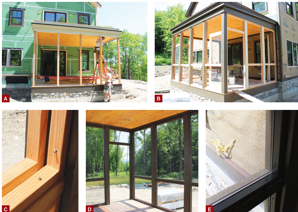
Figure 4. Additional 4x4 posts were installed to frame the openings for the screen panels and doors (A). Prior to screen installation, the trim was painted to match the trim on the rest of the house (B). Fixed (on the exterior) and removable (on the interior) red-cedar stops were added to the openings (C) in preparation for the aluminum screen panels (D, E).
