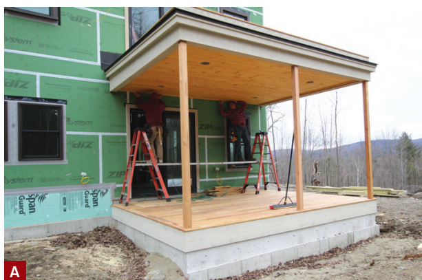
Figure 3. The porch fascia, posts, and eaves were trimmed with Boral TruExterior trim, which is made with fly-ash, a coal combustion by-product, mixed with polymers (A). The porch foundation received a fieldstone veneer finish (B).
