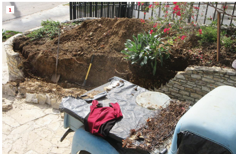
The middle third of a leaning, unreinforced stone retaining wall collapsed during excavation by the homeowner (1).
