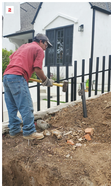
At the street-adjacent curved section of wall, a steel anchor post was driven into undisturbed soil (2). A come-along attached to the steel anchor and a 4-by wall brace pulled the wall back to plumb. Workers reset the 2x4 angled bracing after plumbing up the wall (3).
