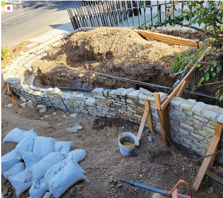
The collapsed portion of the wall was rebuilt using salvaged and new stone (8) . Sheets of 1/4-inch-thick Masonite, 2x4 horizontal blocks, and sandbags were used as wall forms on the shorter curved wall sections (9) .
