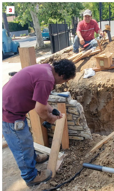
At the street-adjacent curved section of wall, a steel anchor post was driven into undisturbed soil (2). A come-along attached to the steel anchor and a 4-by wall brace pulled the wall back to plumb. Workers reset the 2x4 angled bracing after plumbing up the wall (3).
