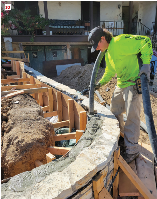
The walls were poured without any blow-outs (10). The author's crew finished off the top of the wall, working around the irregularly shaped capstone (11). The completed retaining wall (12).
