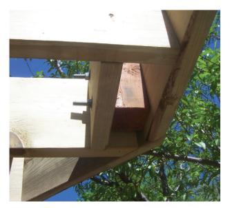
The goal of the new guard-post provisions in the 2021 IRC is to avoid relying on fasteners loaded in end-grain withdrawal as part of the critical guard-post load path. Here, where blocking for the bolted guard-post connection is fastened to the joists, the end-grain connection should be reinforced with additional nails, structural screws, hardware, or some combination of all three.
