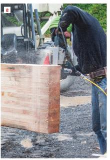
The maximum cut on a  $10^{1/4}$ -inch saw is about  $3^{7/8}$  inches, so cutting through a  $5^{1/2}$ -inch glulam requires two cuts. With the beam positioned on edge and crown up on the forks of the forklift, Kyle Davis cuts vertically from one side (1) and then the other (2).
