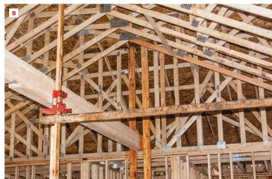
One of the safest ways to lift a beam into place is to first attach the support columns and then lift from the center of the beam with the forklift (6). For larger beams that require more control, the author uses rigging straps (7). If the crew can't use a forklift, they use wall jacks (8), making sure to brace them back to the framing to keep the jack poles straight (9).
