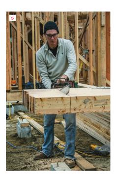
Another way to maneuver a beam is with a "beam wrench," which can be made on site with plywood or OSB scrap (3). This simple moment arm gives the author enough leverage to tip the beam on edge safely and quickly (4). For beam ends that won't be exposed, Kyle makes a first pass with a circular saw and finishes the cut with a chain saw (5), without moving the beam at all.
