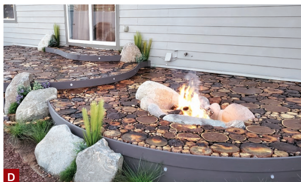
Figure 3. The author cut thousands of log rounds from a variety of sizes and species of wood for the decking (A). During installation, he used screws to hold the larger rounds in place and filled between them with smaller pieces, which were held in place with epoxy (B). After planing and sanding the surface smooth, the author continued to coat the assembly with more coats of epoxy, and wrapped the edge of the deck with composite fascia material (C, D).
