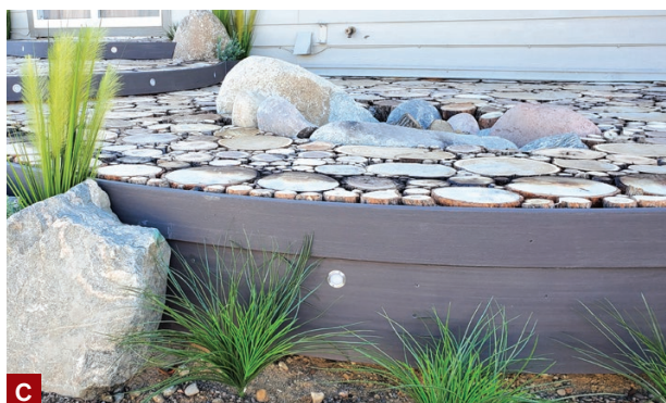
Figure 3. The author cut thousands of log rounds from a variety of sizes and species of wood for the decking (A). During installation, he used screws to hold the larger rounds in place and filled between them with smaller pieces, which were held in place with epoxy (B). After planing and sanding the surface smooth, the author continued to coat the assembly with more coats of epoxy, and wrapped the edge of the deck with composite fascia material (C, D).
