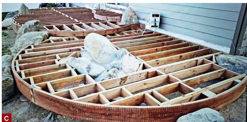
Figure 1. The existing backyard had a small concrete patio, a fire ring, and a few boulders (A). The author removed the patio and repositioned the boulders and fire ring, stabilizing them with concrete (B). The new deck frame was built over new footings and around these features, with a curved rim joist (C).
