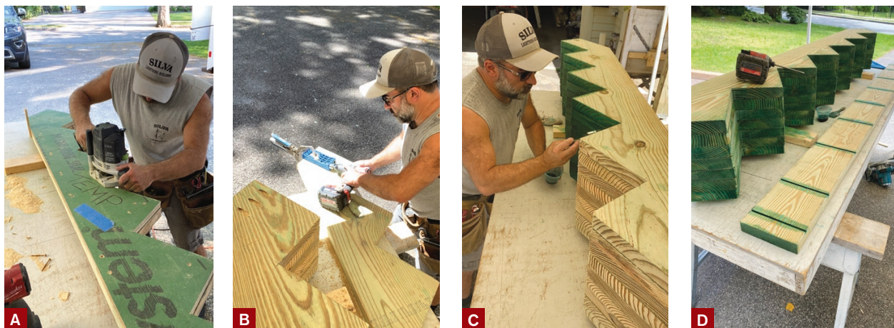
Figure 3. Using a template cut from a double layer of 7/16-inch Zip sheathing, the author pattern-routed the stringers (A). He used a Kreg jig to make pocket holes for mounting screws (B), then screwed the cut stringers together to prevent warping. To prevent rot, he applied preservative to the cuts and notches on the stringers (C) and the landing plate (D).
