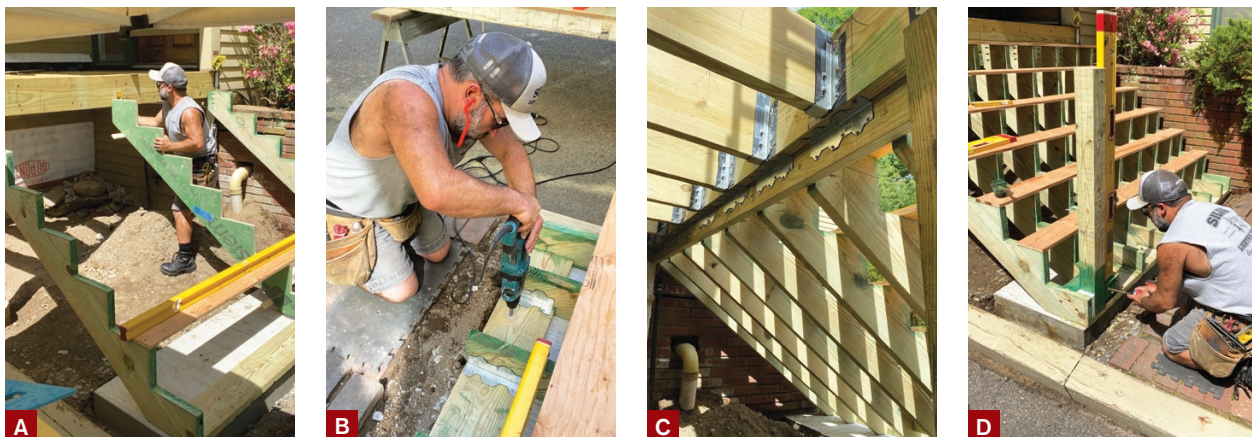
Figure 4. The author installed the end stringers first, then used the template to fine-tune the position of the remaining ones (A). The author used wedge anchors to fasten the plate to the slab (B), and metal angles to attach the dropped header for the stringers to the framing (C). Plenty of blocking was used to reinforce the landing post connection (D).
