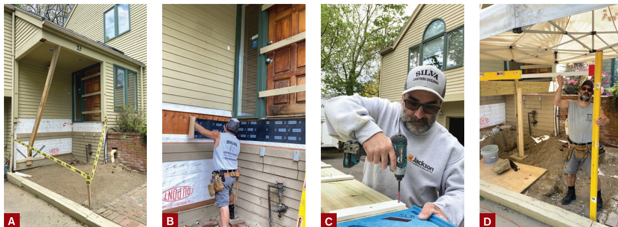
Figure 1. The new porch and stairs had to fit the existing footprint (A). The author covered the wall sheathing with a peel-and-stick flashing membrane (B) and screwed PVC shims to the ledger (C) before installing it. After framing the new porch on temporary supports, the author determined the landing slab's location and elevation (D).
