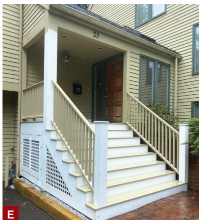
Figure 5. The author used the template that he had made to fabricate the stringers to pattern-route the PVC stringer trim (A), which resulted in a very accurate fit (B). The author also fabricated the post sleeves, stair risers, access door (C), and other porch trim from PVC stock. Along with the 1x4 decking, the railings, balusters, and stair treads were all fabricated from vertical-grain fir that the author prefinished on all four sides with a solid stain (D, E).
