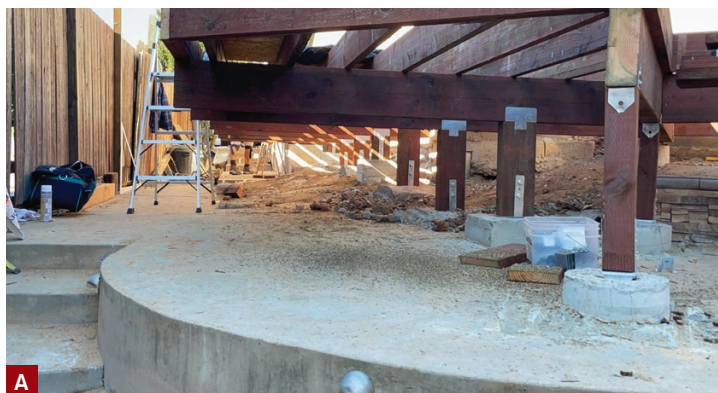
Figure 2. The elevated walkway joists are supported by dropped 4x10 cantilevered beams bearing on 4x8 posts (A). At the house, the beams are anchored to the foundation with upside-down joist hangers to counter uplift (B).
