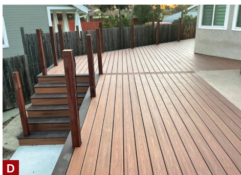
Figure 3. Decking needed to be scribed to fit against the outdoor kitchen's existing stone-veneer wall (A, B). The elevated walkway wraps around the corner of the house (C) and connects with the new main deck (D).
