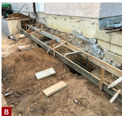
Figure 1. Because of an existing sewer easement (see illustration, above), footings for the elevated walkway along the side of the house could be placed no closer than 5 feet from the municipal sewer line (A, B). Thirty additional piers were also needed to support the main part of the deck, which was designed to extend an existing concrete patio (C).
