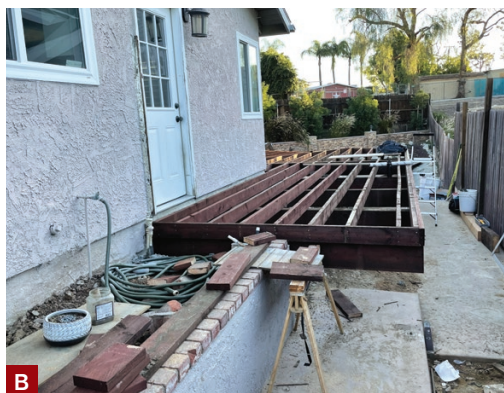
Figure 2. The elevated walkway joists are supported by dropped 4x10 cantilevered beams bearing on 4x8 posts (A). At the house, the beams are anchored to the foundation with upside-down joist hangers to counter uplift (B).
