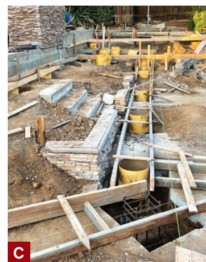
Figure 1. Because of an existing sewer easement (see illustration, above), footings for the elevated walkway along the side of the house could be placed no closer than 5 feet from the municipal sewer line (A, B). Thirty additional piers were also needed to support the main part of the deck, which was designed to extend an existing concrete patio (C).
