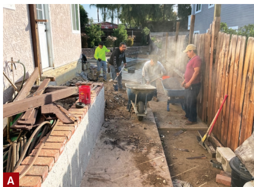
Figure 1. Because of an existing sewer easement (see illustration, above), footings for the elevated walkway along the side of the house could be placed no closer than 5 feet from the municipal sewer line (A, B). Thirty additional piers were also needed to support the main part of the deck, which was designed to extend an existing concrete patio (C).
