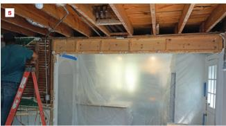
Plumbers over the century had done a good job of carving up floor joists (4). The span and width of this undermount header (5) required a double LVL, but the remodelers who installed it to open up the room to the kitchen had used a double 2x12 instead.
