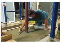
At the top of the wall section described above, the pencil line (13) shows the position of a laser before the beam is jacked into position in the basement (14). When the beam is level, the wall has been raised more than an inch (15). Steel shims are placed between the new beam and the old basement girders (16). A new footing is prepped (17) and poured (18) for the new column.
