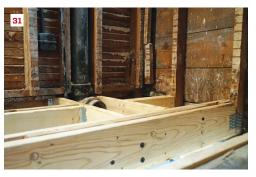
At one end of the flush beam, the load path from beam to window header to full-height jacks is complete (28). At the other end, the flush beam has full bearing on a corner column (29) that bears directly on the new steel beam that spans the girders in the basement. To complete the job of reinforcing the floor system, the joists hacked up by plumbers are headed off (30, 31).
