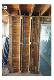
Ernesto Bonilla cuts flooring nails (8) so sister joists will fit tight to the existing ones. He and Toby Bonilla roll in sister joists (9); a screw and hammer help pull the sisters flush to the bottom edge of the existing joists (10). Blocking is key to stiffening the floor (11). The studs in this critical wall section (12) had bowed and are reinforced before any jacking is done.
