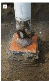
In this joist bay (6), a new steel beam will be installed perpendicular to this basement girder. (It will span to another girder that runs parallel to it). The column supporting this girder had almost no footing (7).
