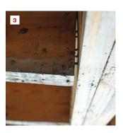
This flush beam in the second floor had no bearing on one end, only nails loaded in shear into a ledger (1). The ledger was partly carried by cripple studs, but the header supporting these cripples had no support (2). No joist hangers supported the joists carried by the flush beam (3), and the end nails had pulled away as the beam, which was overloaded on one side, had rolled.
