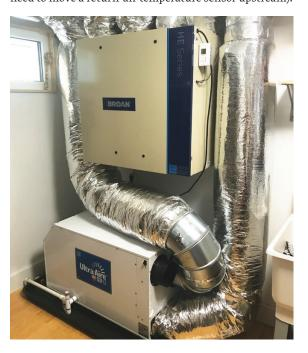
Most ERVs like this one (upper piece of equipment) have ports for standard 4- or 5-inch ductwork. Note that this system includes the indoor coil (lower piece) for a dedicated dehumidifier, which will be needed in most locations to address latent loads.
