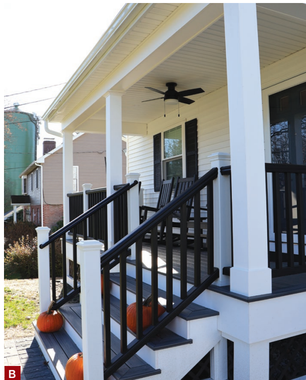
Figure 4. The deck's three site-built "laminated" 6x6 rough posts were finished with PermaSnap composite column wraps. Here, the 1/2-inch-thick white composite trim is temporary taped while its adhesive cures (A). A Trex composite guardrail system encloses the completed porch (B).
