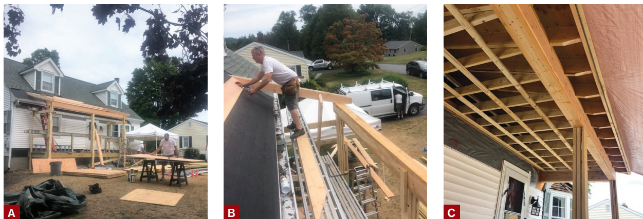
Figure 2. Crew members framed the new 7-foot-by-18-foot porch (A), tying it to the main roof (B). The upper porch was framed with site-built “laminated” 6x6 posts supporting a triple 2x10 girder, 2x8 rafters, and 2x6 ceiling joists (C).
