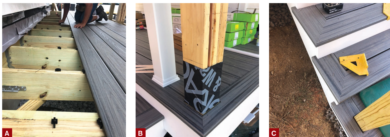
Figure 3. Hidden fasteners were used to install the Trex porch decking (A), while color-matched trim-head screws were used to fasten the picture-framed perimeter edge boards (B) and stair treads (C) to the framing.
