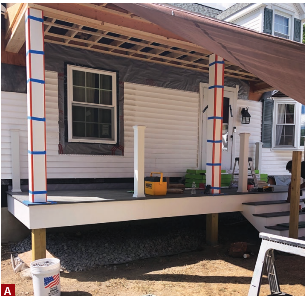
Figure 4. The deck's three site-built "laminated" 6x6 rough posts were finished with PermaSnap composite column wraps. Here, the 1/2-inch-thick white composite trim is temporary taped while its adhesive cures (A). A Trex composite guardrail system encloses the completed porch (B).
