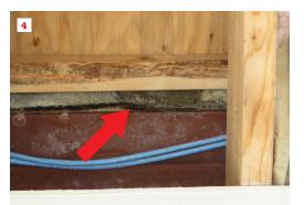
After 10 minutes, water appeared inside the house at the bottom edge of the felt WRB, which terminated at steel angle shelf (4). Removal of a stone confirmed that through-wall flashing had not been installed (5).
