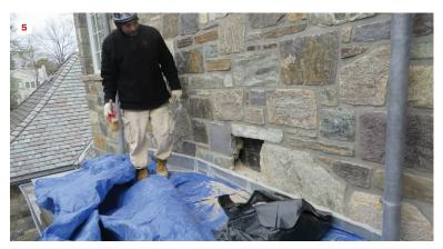
**New clients** had a problem with their existing home: A projecting bay would leak at the ceiling during heavy rain. It had happened often enough that they had removed the drywall and insulation, ready—we imagined—to place buckets below to catch any incoming water.
