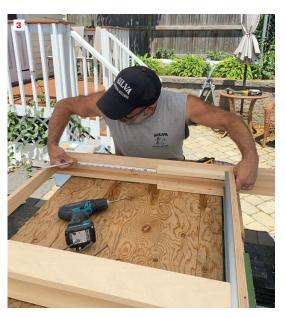
The fully assembled Johnson Hardware 30-inch pocket-door unit was ready to install in the rough opening ... except for one problem: It was 8 inches too wide (1). To trim it to fit, the author started by unscrewing the aluminum track from the door header (2) and marking the new width required for a 26-inch door on the header (3).
