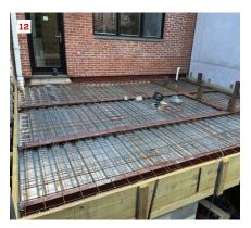
Blocks are fitted around the beam ends to form pockets (10), and short, intersecting I-beams are added between the main beams (11). These short beams will support the square tubing stub-outs that will connect to the fire escape. The deck, which will support the fire escape and serve as a patio, is ready to be poured (12).
