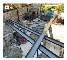
With the basement-level block walls up, the crew receives the individual pieces of steel C-channel for the beams, threading them through a front window (4) and carrying them through the house (5). The lengths of C-channel are placed atop the block walls to be fabricated into beams (6).
