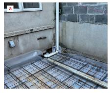
Before work began, the building stepped back on the second and third levels. Additions on the two levels will align with the brick wall of the main level (1). With the back patio demolished, block work begins (2), and an extension of the basement-level slab is prepped for the pour (3).
