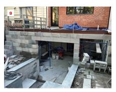
To create the beams, the steel fabricator spot-welded and bolted the C-channel together (7). Angle iron to support the corrugated steel decking was bolted to the C-channel, and the completed beams were painted with red oxide primer (8, 9).
