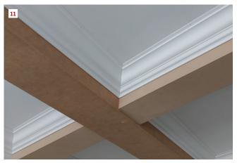
A bead of hot glue adds strength to the outside miter after the joint is preset. By gluing the miter on the ground, I find it easier to get the right fit (9, 10). Installed and ready for paint, crown always makes an impression (11).
