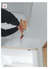
With the saw set at a 33.9 bevel and 31.6 miter on the table, we can cut the crown on the flat (5). Alternatively, hold the crown "in position" against the line drawn on the fence and set the bevel at 0 and miter at 45 (6). By holding a jigsaw at the opposite angle of the miter, you can make an ideal back-cut (7). The aptly named "tappy" block helps adjust the crown into place (8).
