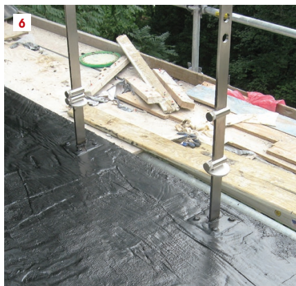
Preinstalled posts. The bases of these posts for glass railings needed to be bolted to the masonry deck (4, 5). The bases were waterproofed (6) and finished with stone and round escutcheon plates (7).
