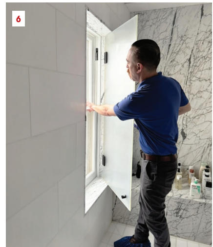
One of the last components to install is the first line of defense against splashing water: The author's company has the shower glass subcontractor fabricate hinged glass panels to cover the window (5, 6).
