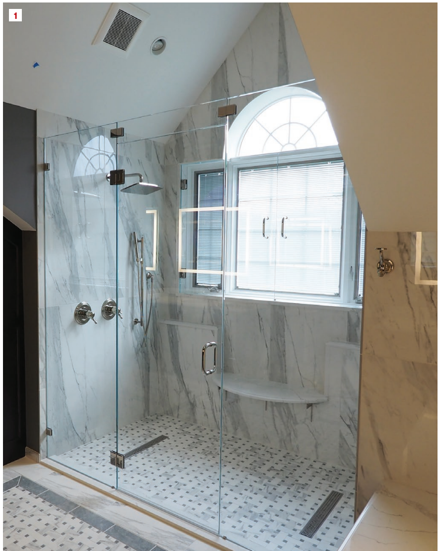
Windows in showers are valued by many clients, but they present a moisture risk from both splashing water and condensation. That requires multiple lines of defense.
