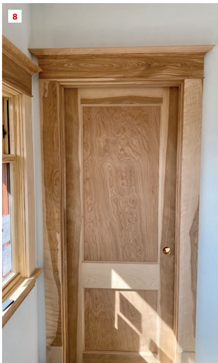
To case around custom birch doors, the author used yellow birch with a mix of sapwood and heartwood, going for a "wild" look as requested by the client (8). The ray fleck visible in quartersawn oak (most prominent on the casing and door on the right) is often called "tiger stripes." (9).
