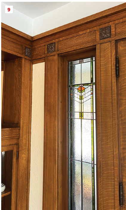
To case around custom birch doors, the author used yellow birch with a mix of sapwood and heartwood, going for a "wild" look as requested by the client (8). The ray fleck visible in quartersawn oak (most prominent on the casing and door on the right) is often called "tiger stripes." (9).
