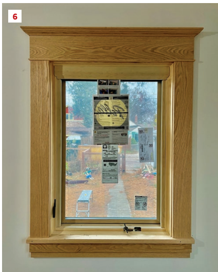
Another example showing a variation in how the grain of a head casing can be centered over the window (6). One leg of any corner molding will have flat grain (in this example, it's the horizontal leg on top), and the other leg will have vertical grain (7).
