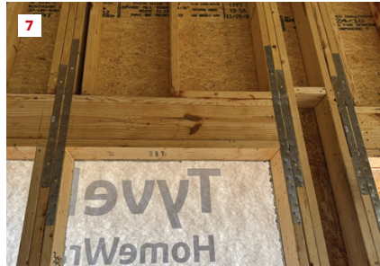
6 Gable-end trusses were tied to the gable-end walls with metal straps. To meet Fortified Gold, the size, frequency, and nailing needed to be specified by an engineer.
