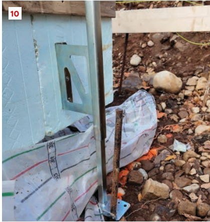
Adjusting for elevation and level across the block is done in unison on bracket pairs (9). A ground pin to hold the HD bracket is driven into the bedrock just below the soil (10).
