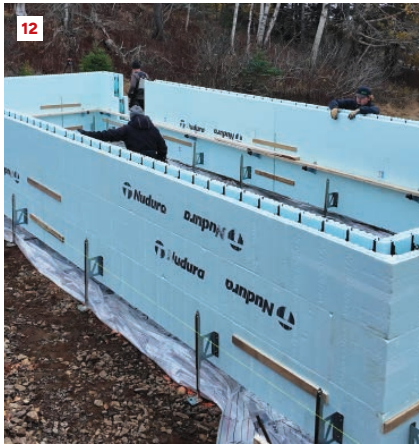
With each block course and bracing attachment the crew confirm square (11). Note how the Fastfoot material is moved out from under the HD bracket (12).
