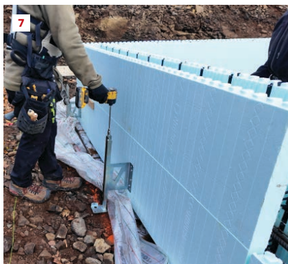
This is an example of a stacking or marriage joint. It is bound with strapping and glued (6). The HD bracket can be raised or lowered with a drill/driver or socket wrench (7). Checking for wall straightness is done with each adjustment and new wall course (8).
