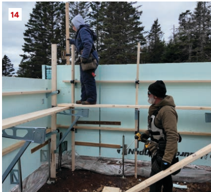
This is the "Zont" bracket to hold walers and strongbacks. The plastic cam locks them in place (13). The foldable "Zat" (14) creates the walkway with guardrail when attached to the bracing. It also provides the attachment for the "Zuckle" wall aligner hardware.
