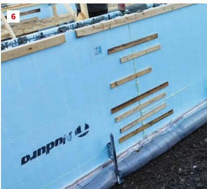
This is an example of a stacking or marriage joint. It is bound with strapping and glued (6). The HD bracket can be raised or lowered with a drill/driver or socket wrench (7). Checking for wall straightness is done with each adjustment and new wall course (8).
