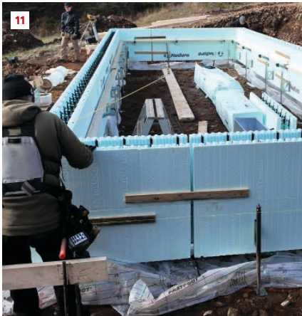
With each block course and bracing attachment the crew confirm square (11). Note how the Fastfoot material is moved out from under the HD bracket (12).
