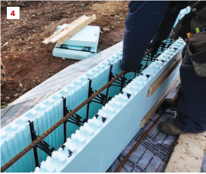
Here you can see where rebar is snapped into the ICF webbing per the plan's spec (4). HD brackets are attached in pairs (one outside, one inside) to the ICF block (5).
