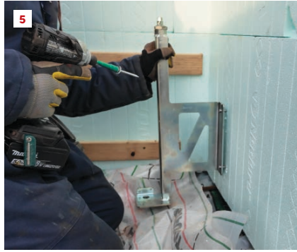
Here you can see where rebar is snapped into the ICF webbing per the plan's spec (4). HD brackets are attached in pairs (one outside, one inside) to the ICF block (5).
