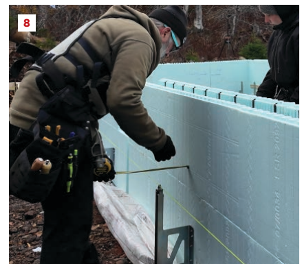
This is an example of a stacking or marriage joint. It is bound with strapping and glued (6). The HD bracket can be raised or lowered with a drill/driver or socket wrench (7). Checking for wall straightness is done with each adjustment and new wall course (8).
