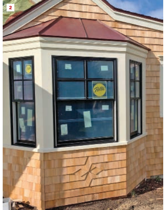
The author devised two different corner treatments using copper flashing that he has since used on a number of exteriors—an open square corner (1) and a single fin (2).
